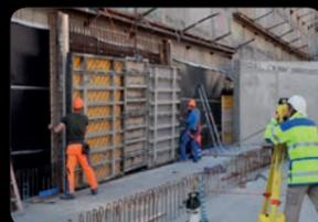
iCON builder 60 can be also used as one-person station for checks, such as tie distances, clearance or verticality
