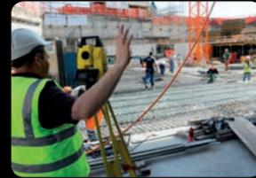
Layout points on blinding layer such as pipe insert or cut-outs before pouring concrete
